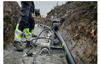
HV Cable laying Works
