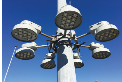
High Mast Works
